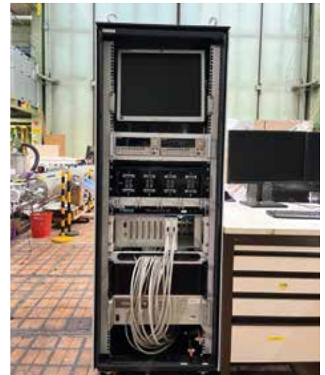
Fig. 8: Mobile measuring rack for the acceptance test of the quench sample
