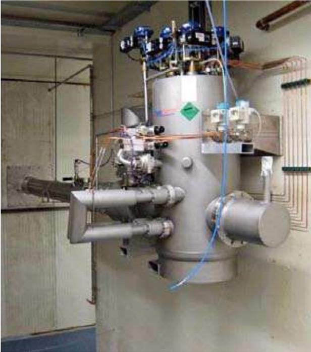
**Fig. 6: Cryotransfer line; the valve box for the WGTS was installed at the TLK in 2008.**
