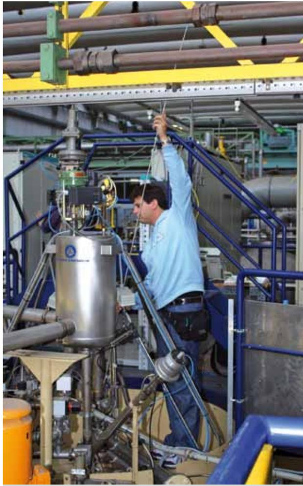
*Fig. 8: Implementation of a new temperature sensor in the 5000-liter tank of the 300-W facility.*
