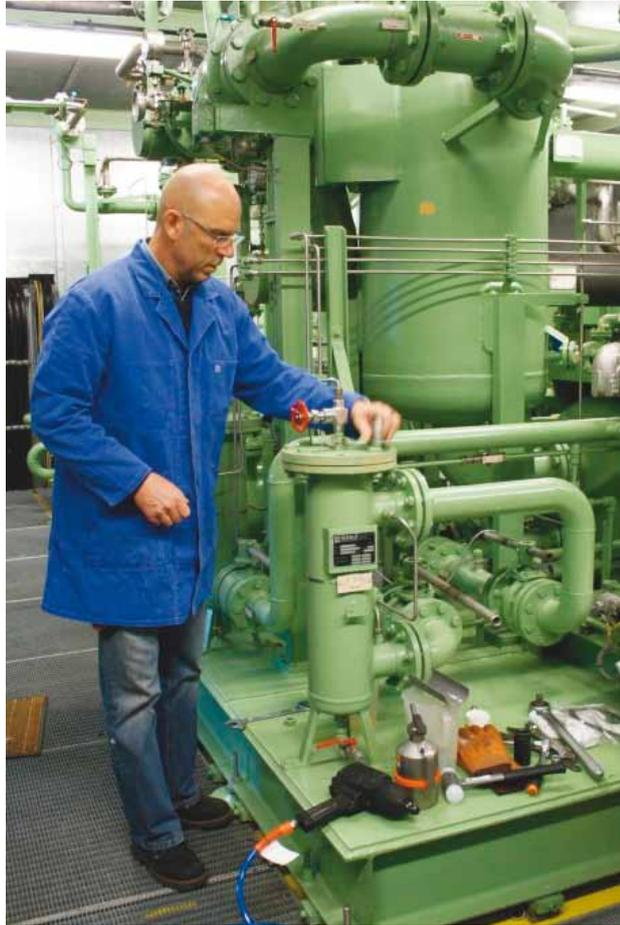
*Fig.7: change of the oil filter at the oil-sealed screw compressor of the 2 kW-refrigerator.*
