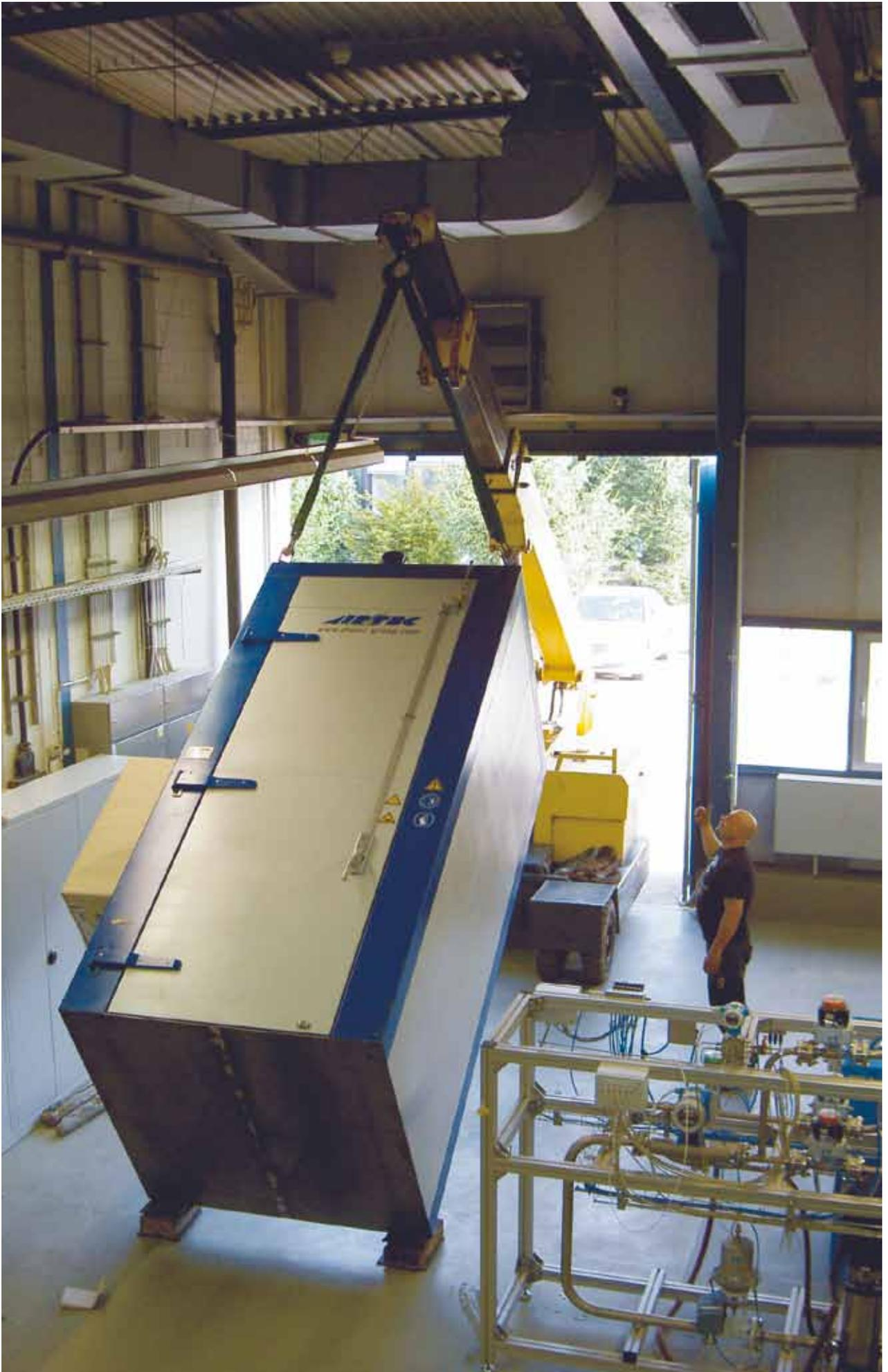
*"Installation of the heating oven for the new coating facility".*
