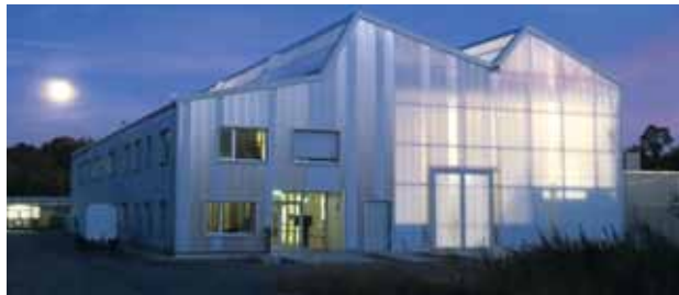
Fig. 10: Exterior of the new laboratory building 668 hosting the microgrid and the Power-Hardware-in-the-Loop laboratory.
