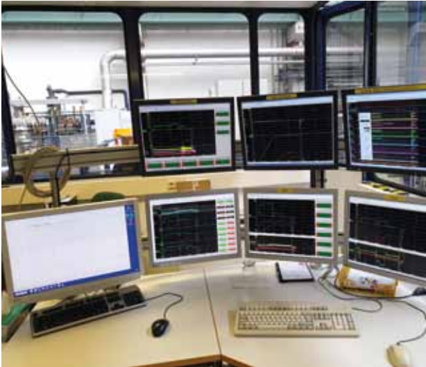
Fig. 17: Newly upgraded control system for magnet monitoring with quench detection for the independent current circuits of the NbTi-, NbSn- and HTS-magnet subsystems.
