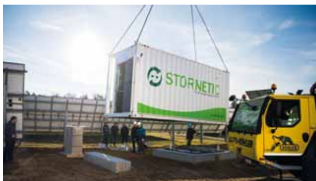
Fig. 11: Installation of a 60 kW, 3,6 kWh flywheel energy storage system at the Energy Lab 2.0 site of the KIT.
