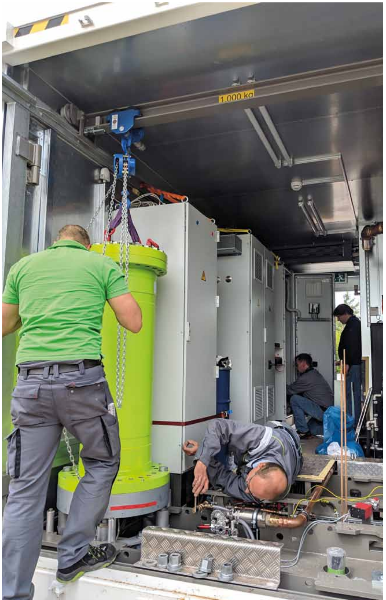
Installation of a 60 kW-3.6 kWh flywheel mass storage for the Energy Lab 2.0 at KIT
