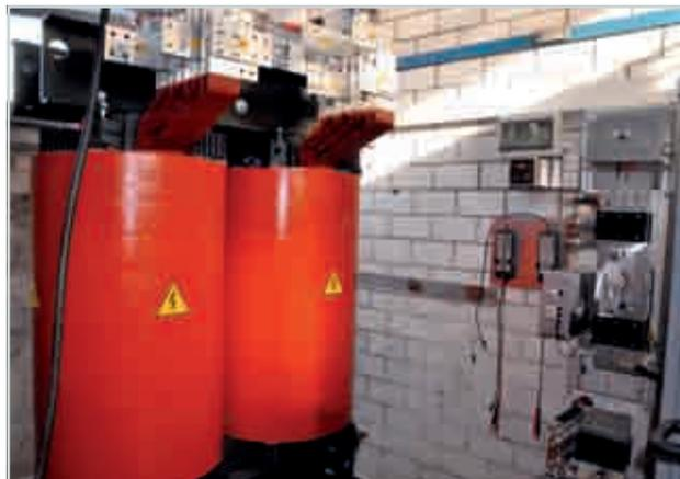
Fig.9: New single-phase 1.2-MVA continuous-load short-circuit current test facility of ITEP.
