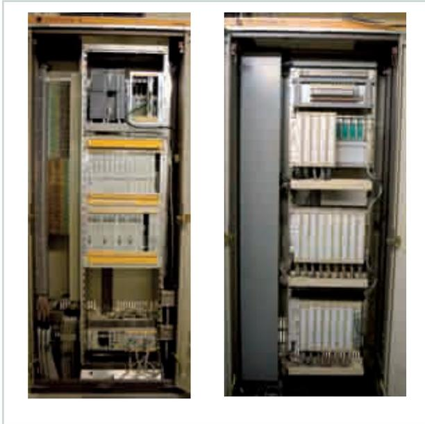
Fig. 7: Cabinets for Teleperm-AS488 and Simatic-S5.
