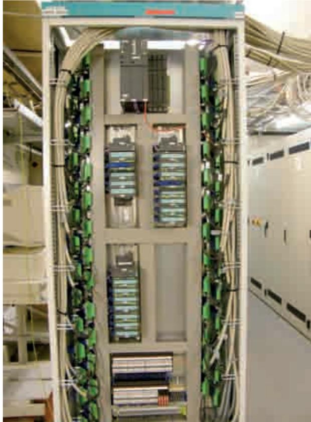
*Fig. 10: New Simatic PCS7-AS417 control unit with analog and digital I/O peripheral subassemblies.*
