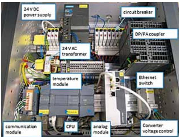
Figure 3: Hardware of the temperature control unit.
