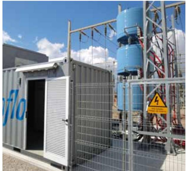
**Figure 4: ECCOFLOW current limiter at the ENDESA transformer station, Palma de Mallorca.**
